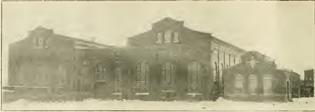
NORTH END OF LOCOMOTIVE SHOP, WITH MACHINE SHOP IN CENTER AND CLEANING-PIT HOUSE AT RIGHT.
